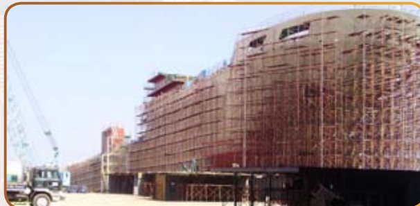
PHOTO - HULL 157 UNDER CONSTRUCTION
